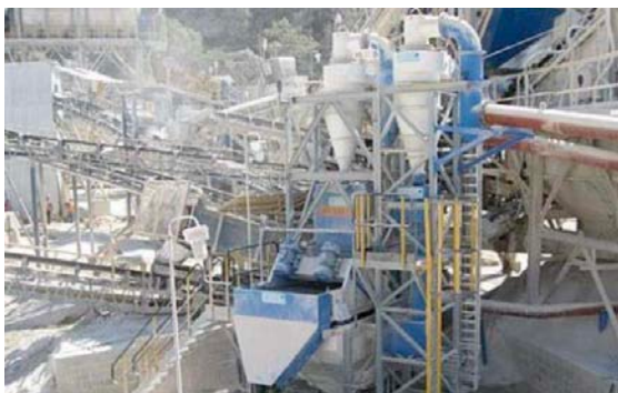
Integration of two cyclones for washing and classification processes in a quarry site
