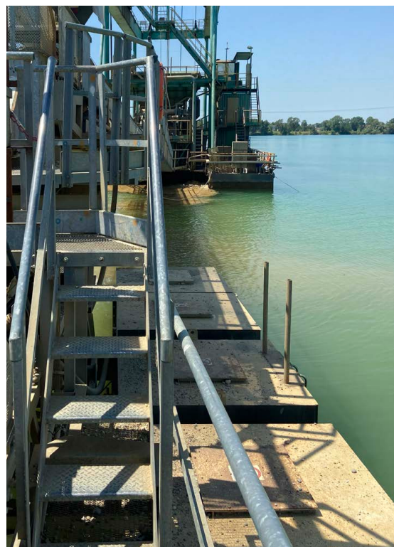
Aggregates extraction with a dredger. Holcim – Italy
