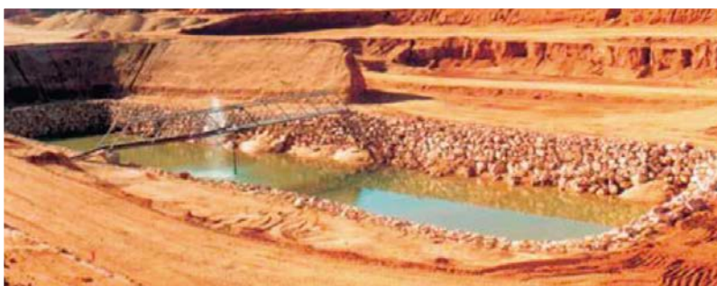
Cleaning water pond – Sand and gravel pit – El Tomillar site – Hormisoria, S.A. - Spain
