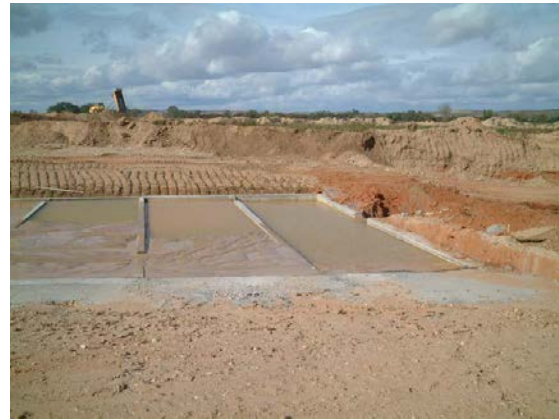
Sludge concrete ponds – Sand and gravel pit – FdA – Spain
