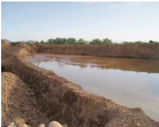
Small sludge dam
