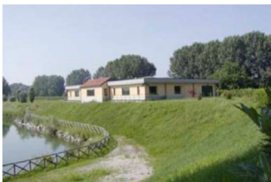
Sand and gravel pit – La Loggia site – Zucca e Pasta - Italy
